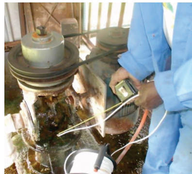
Figure 6: Measuring the Water Level with a water level meter 3
